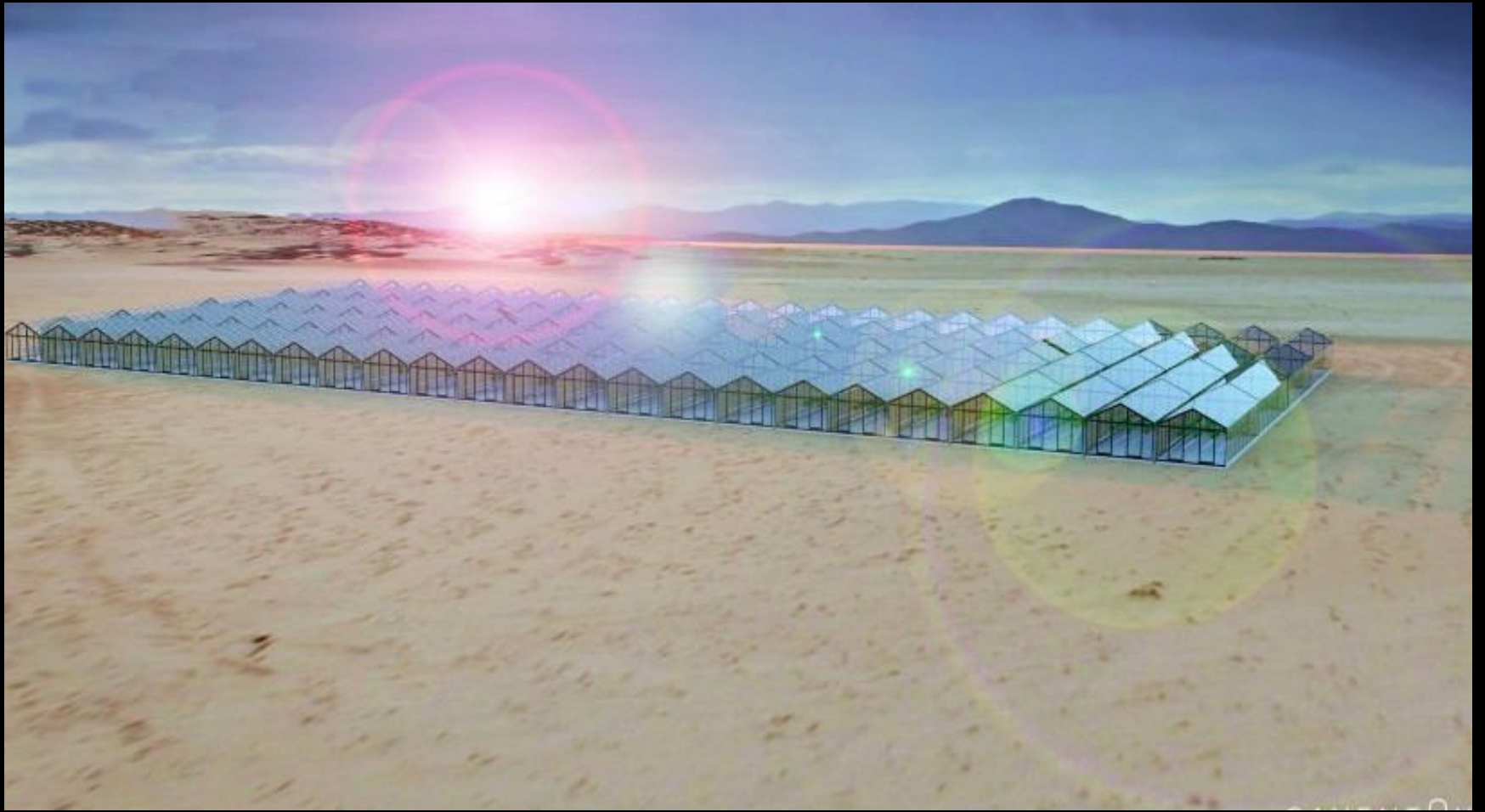
Power Plant, Caventou
