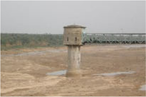
French wells for recharging the ground water level of the river bed
