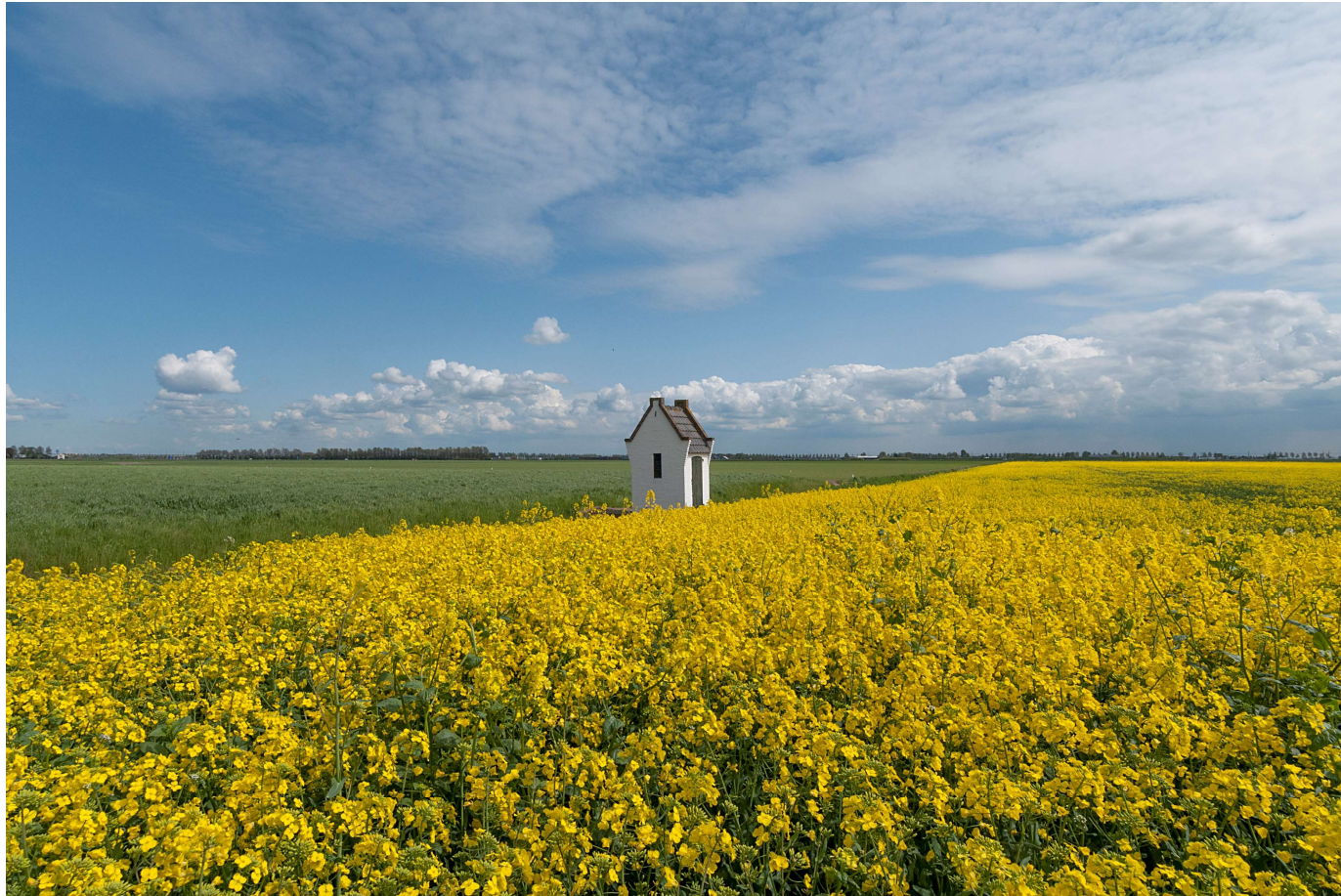
Small dewatering house near Nieuw-Vennep
