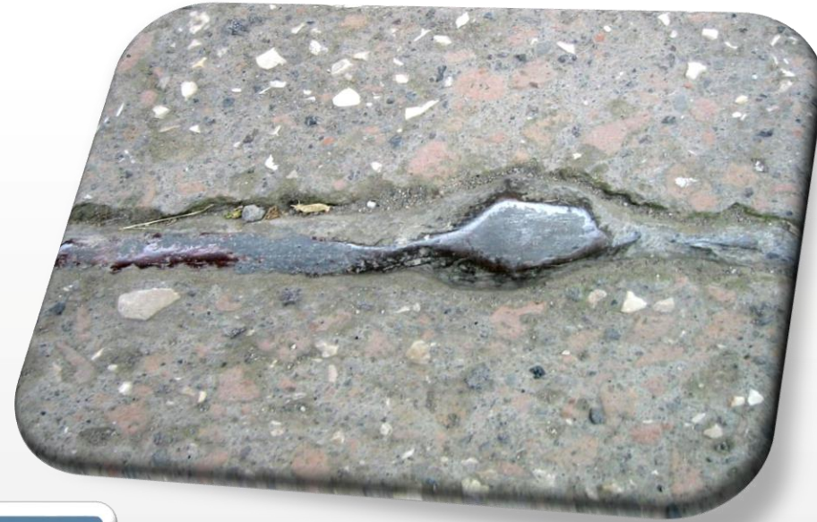
Roman pipe still built-in pavement – outdoor archaeological site Cluj-Napoca
