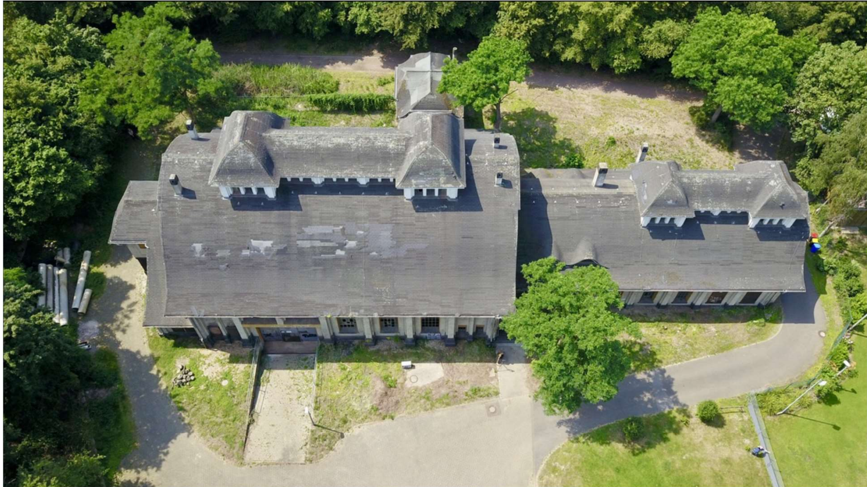
Das Klärwerk Krefeld, Rhineland, Germany, 1908 one of the oldest wastewater treatment plants.
